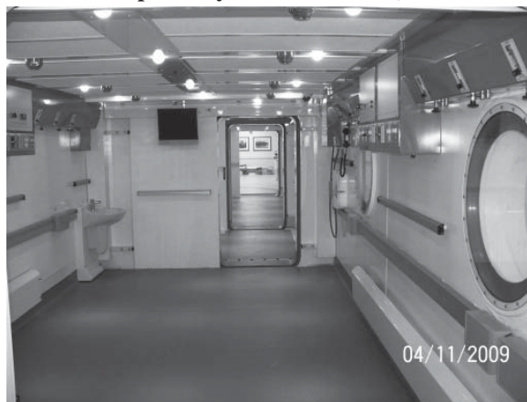
Figure 2 A chamber designed to treat multiple patients (The Karolinska Institute, Stockholm; photo by Peter Kronlund)
